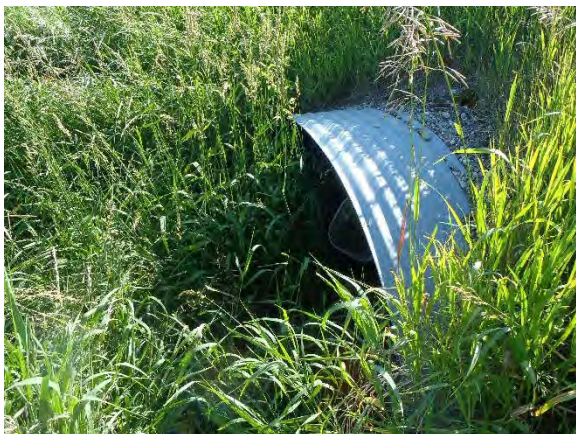
Photo 3- Downstream end of CSP Culvert under Hwy 7
